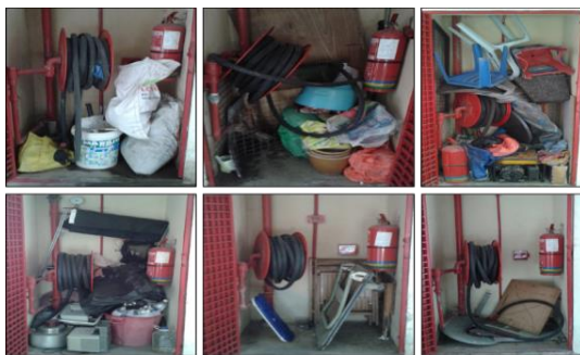
Figure 8: Potential fuel sources in the fire-fighting equipment room
