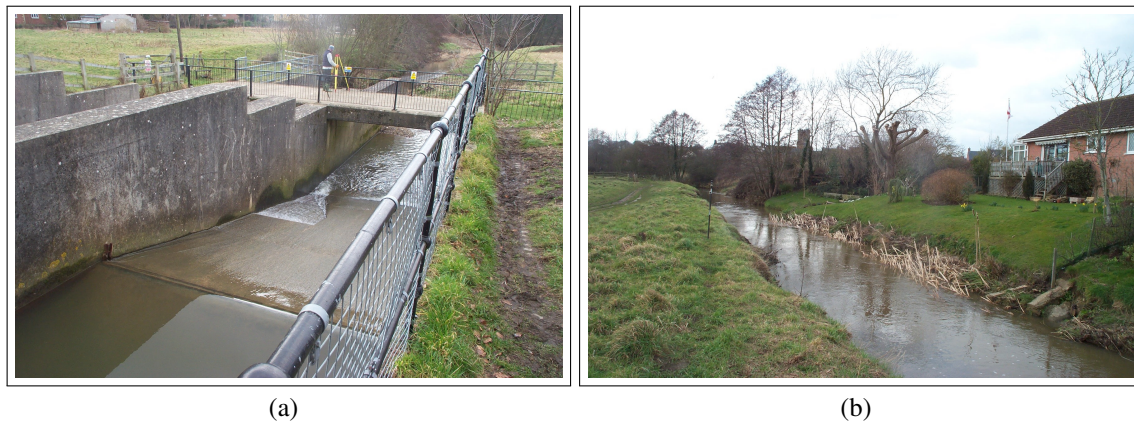
Figure 6.1 (a) Asker River downstream flow gauge (FG1 in Figure 6.2 (a)) and (b) location of surface drainage outfall (DO1 in Figure 6.2 (c)) [looking downstream]
