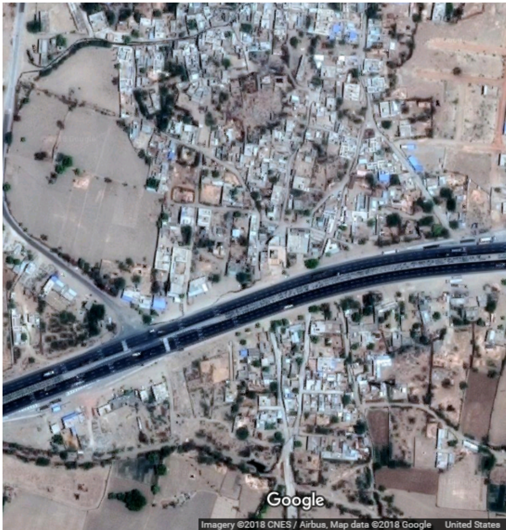
Figure 8: A six-lane national highway passing through a village (Source: Google Earth snapshot)
