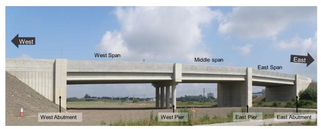
Figure 3.1 Nine Wells Bridge used for the scour simulation (courtesy of Tina Schwamb)
