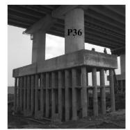
April 2009 (piles exposed around 4.5m)July 2009 (piles exposed around 7.5m)Figure 2.20 Foundation exposure of Hsichou Bridge, Taiwan (Ko et al., 2010)
