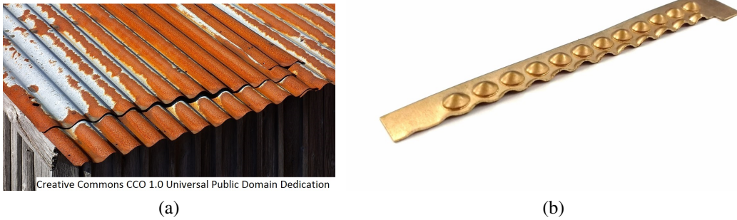
Fig. 2.2 (a) The undulating cross-sectional profile of a corrugated sheet greatly increases the bending stiffness in one direction by increasing the effective structural depth. (b) The cross-sectional profile of a dimpled sheet is also undulating, but unlike a corrugated sheet it undulates in the perpendicular direction also.
