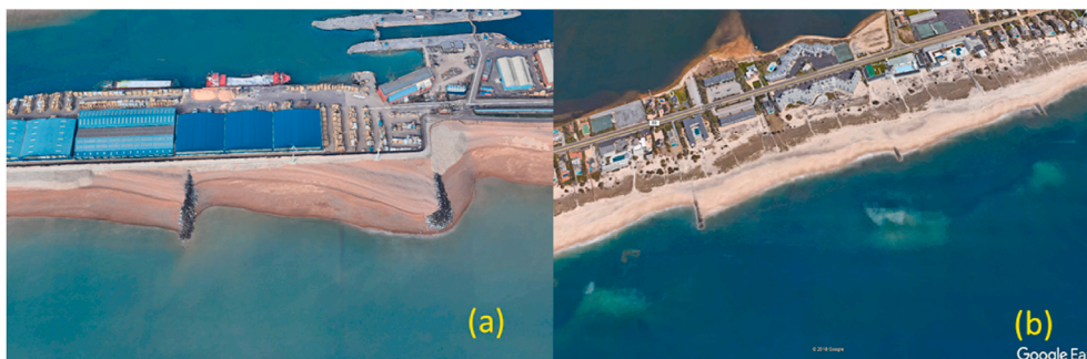
Fig. 3. (a) The terminal groyne syndrome occurring in Southwick beach in West Sussex where the net littoral drift is from left to right. (b) The same phenomenon is observed in Westhampton beach in New York where the net littoral drift is from right to left (photos extracted from Google Earth).
