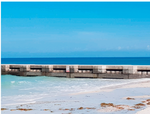
Fig. 19. The innovative groyne design concept that allows for adjustment of groyne permeability by adding/removing pre-cast concrete blocks (photo: Cortez beach, Florida).
