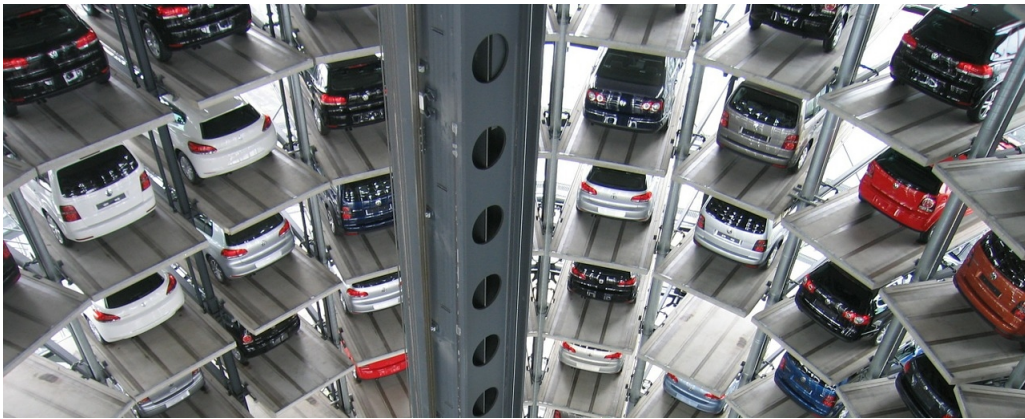
Figure 2.1: Automated parking garage with vehicle elevator [6].
