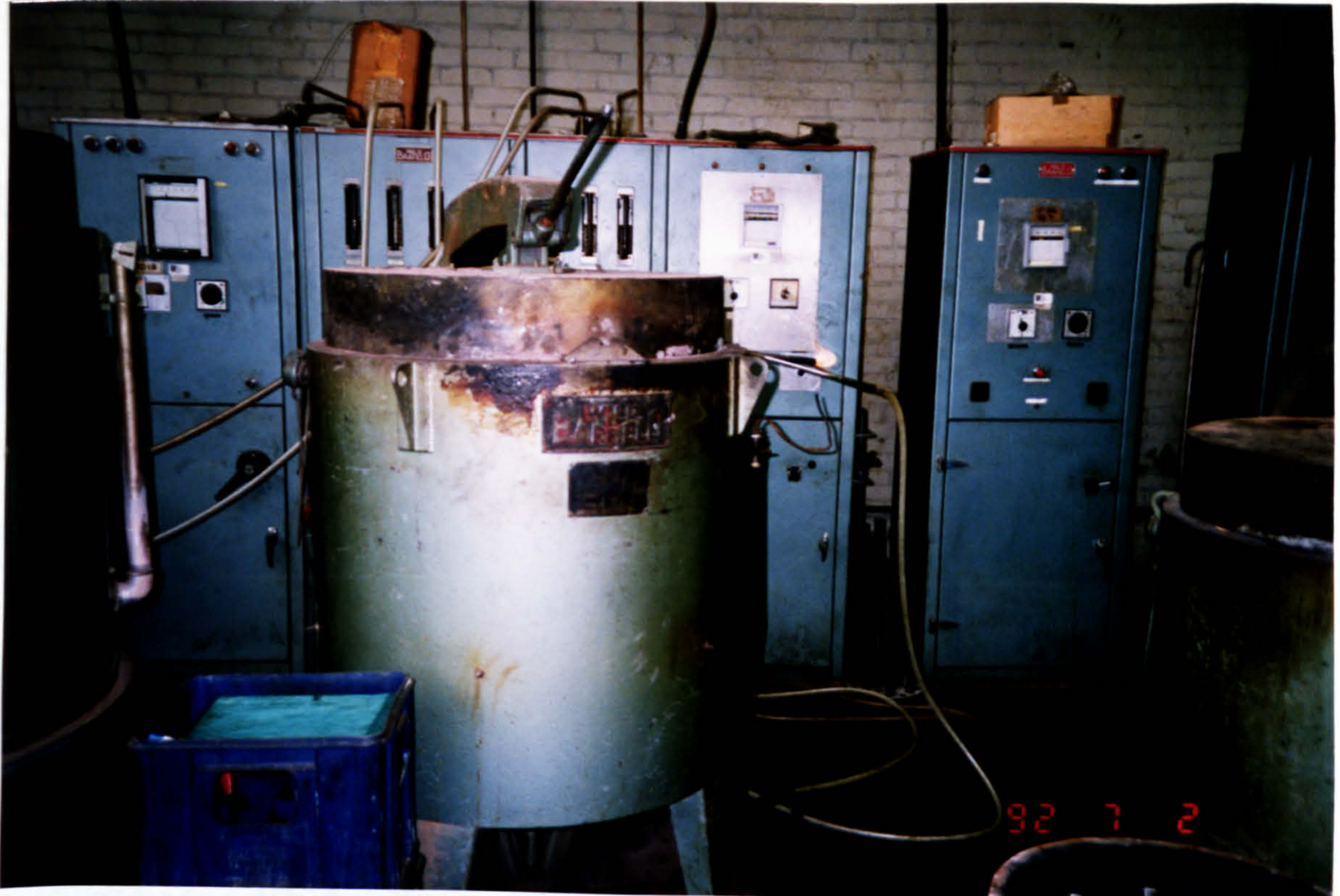
(a) Gas nitriding furnace
