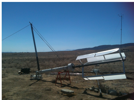
(a) Turbine lowered during rotor installation
