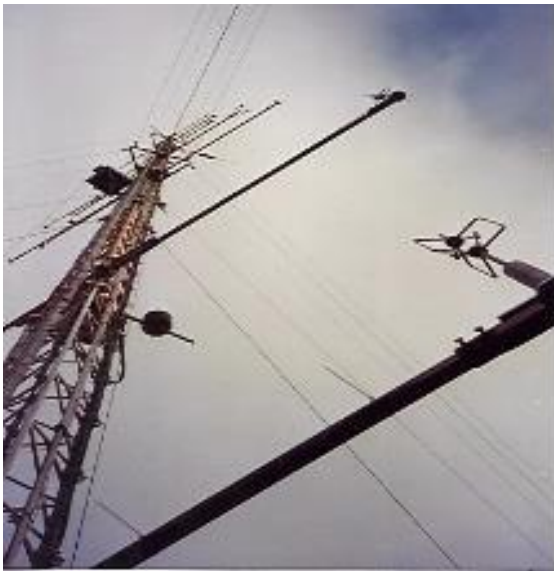
Figure 6. Picture of the 48 meters-high mast.
