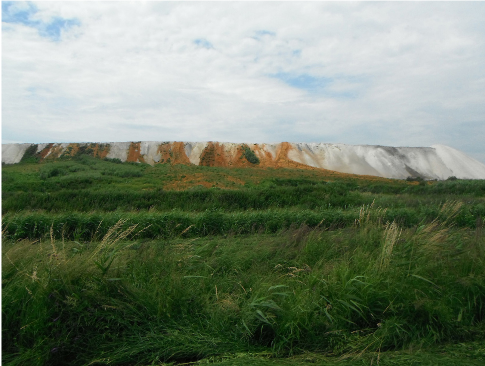
Figure 2. Phosphogypsum stack in Police
