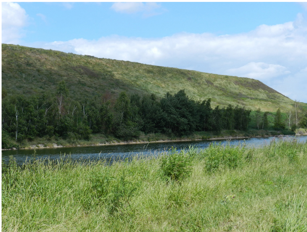
Figure 1. Phosphogypsum stack in Gdańsk
