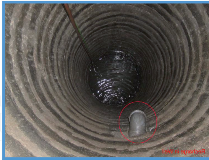
Figure 4. Dug well groundwater recharge structure.
