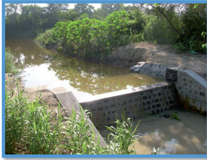
Figure 3. Check dam for surface water harvesting.
