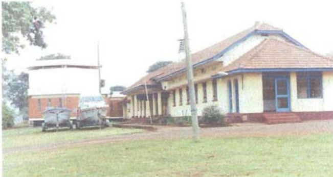
Laboratory (right) and conference (left) blocks at the headquarters of the Fisheries Resources Research Institute (FIRRI), Jinja
