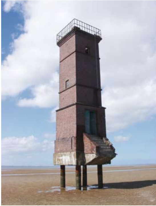
3.7 > The old lighthouse on the East Frisian island of Memmert once stood in the dunes, but was washed out by erosion over the course of decades.
