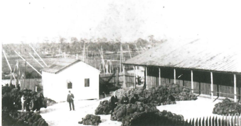
Figure 4.19 View from west side of the old wood sponge exchange with the Anclote River in the background.
