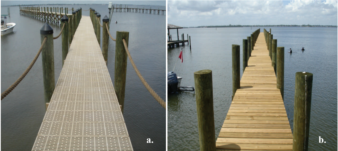
Figure 1. Light transmitting (a) and planked (b) docks.
