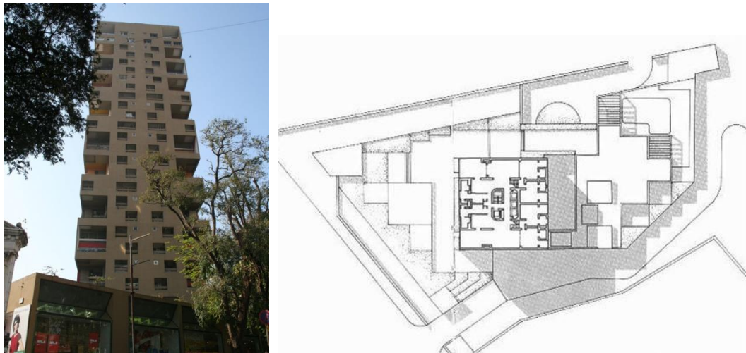
Figure 2: Kanchanjunga Apartments (general view and site layout).
