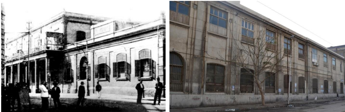
Figure 3: Left: old photo of the Bourse of Minet El-Bassal, designed by P. Avoscani (Awad 2008, 78) and Right: new photo of the Bourse of Minet El-Bassal. (Source: authors, 2012).
