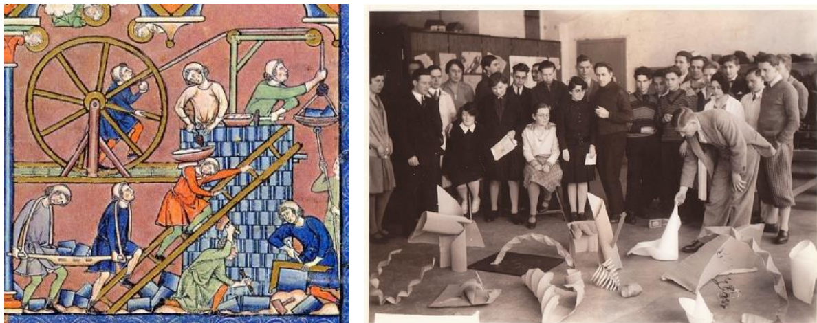
Fig. 1 The contrast between the practical teaching in a high medieval construction site and the design studio of Josef Albers with students of the preliminary course in 1928 in a critique at the Bauhaus in Dessau illustrating the progressive changes in history (photos from Maciejowski Bible and Otto Umbehr)
