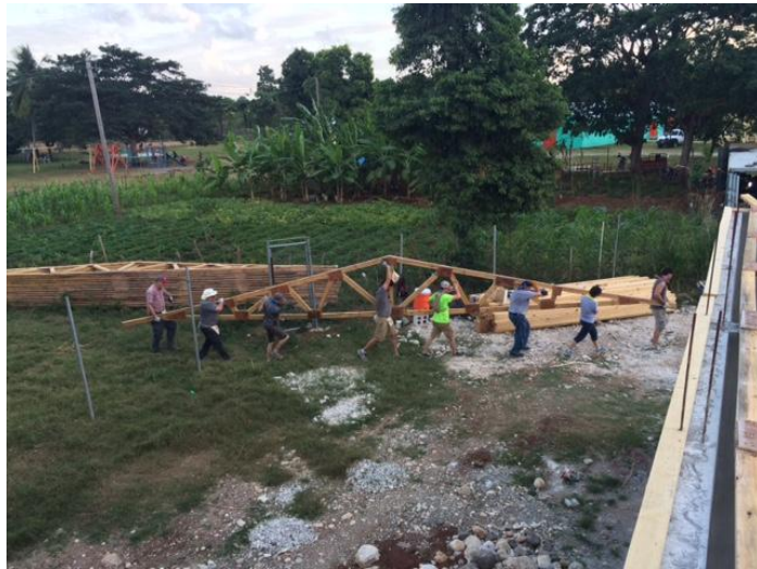
Fig. 22 Volunteers and workers working on site
