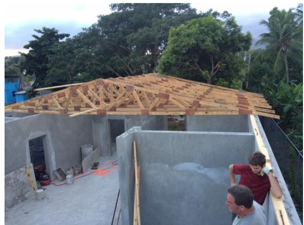
Figs. 23,24 Roof assembly. Volunteers and workers on Site. January 2016.
