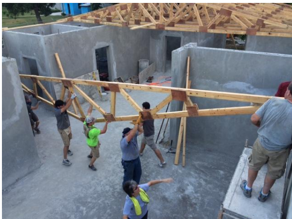
Figs. 23,24 Roof assembly. Volunteers and workers on Site. January 2016.
