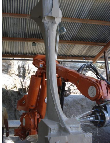
Fig. 7 Robot fabricating a stone component for one of the facades of the Temple of the Sagrada Família.
