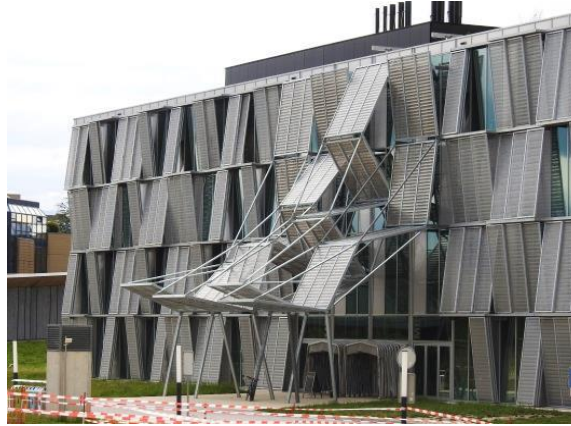
Fig.12: ME Building (Laboratory of Biomaterials) in EPFL Campus in Lausanne, Switzerland. It is an example of emphasizing the entrance approach by the design of a kinetic canopy, designed by Dominique Perrault Architecture - Source: Photographed by the author, 2019
