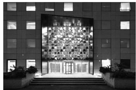
Fig.7: Bianchini Office Building, Italy Source: Archilovers
