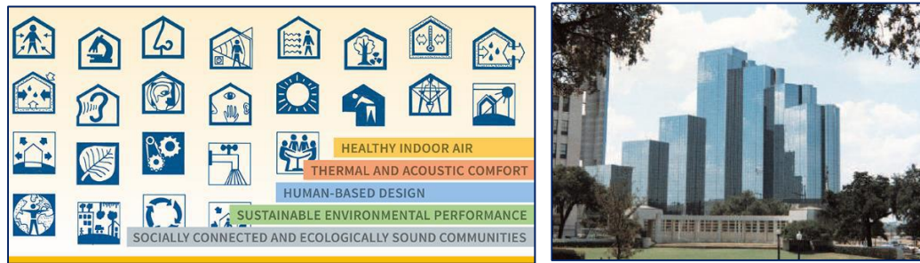
Figure 2: Left: The 25 Guiding Principles of Building Biology. Source: IBN (2018) Right: Dallas, Texas, USA: Hyatt Regency Hotel (1970s): Clad of reflective glass that requires conditioned air to offset heat loss and gain daily and seasonally. Source: Thomas (2002)
