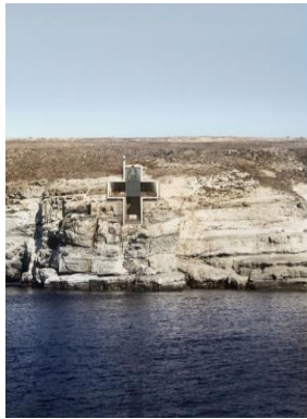
Fig.14: Day shot of the building
