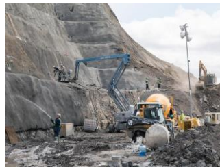
Fig.2: Construction equipment on difficult topography
