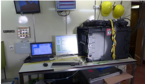
Figure 30: Atmosphere intake system (AIS) with the Picarro measurement control computer (right computer screen) and the OFOP data logging computer (left notebook) in the wet-lab.
