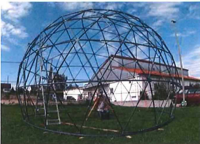
Left: Test assembly of the support structure. Note the modular foundation ring at the base. Correct dimensions were validated using a theodolite. Right: Rear projection test without the inner canvas. Note the projector (on boxes) and the evacuation nozzle at left. The dome rests on 10 vertical metal struts of 2m length. The projection (one channel active) is calibrated for 180° FoV. All photos by and/or courtesy the author.
