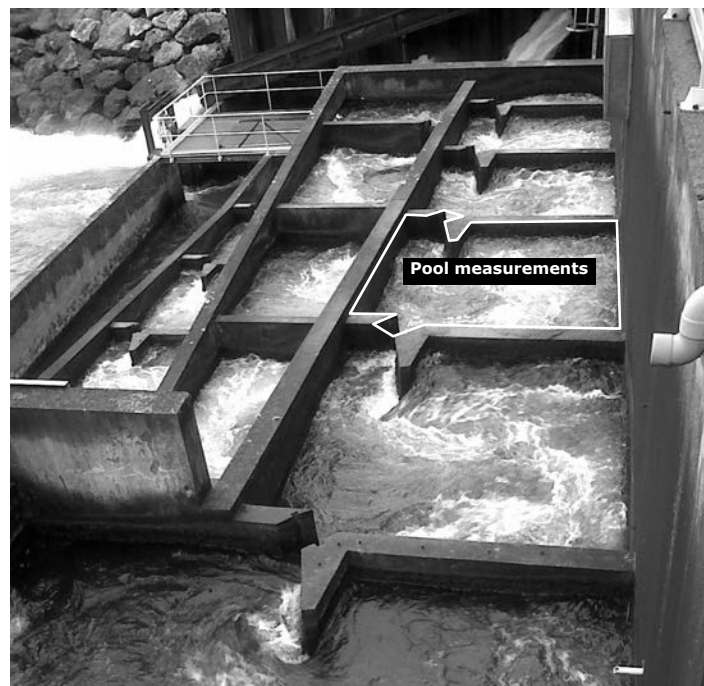
Figure 1. Vertical slot fishway of the hydroelectric power station of Pardies on Gave de Pau River.
