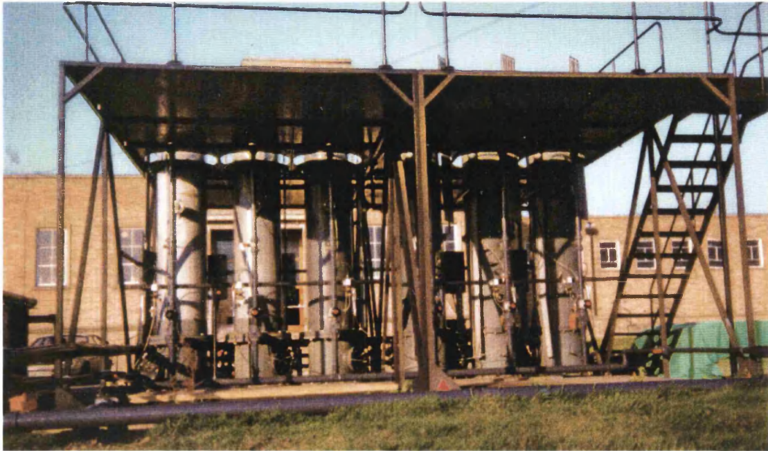
Figure 3.3. The pilot plant under construction in 1989.
