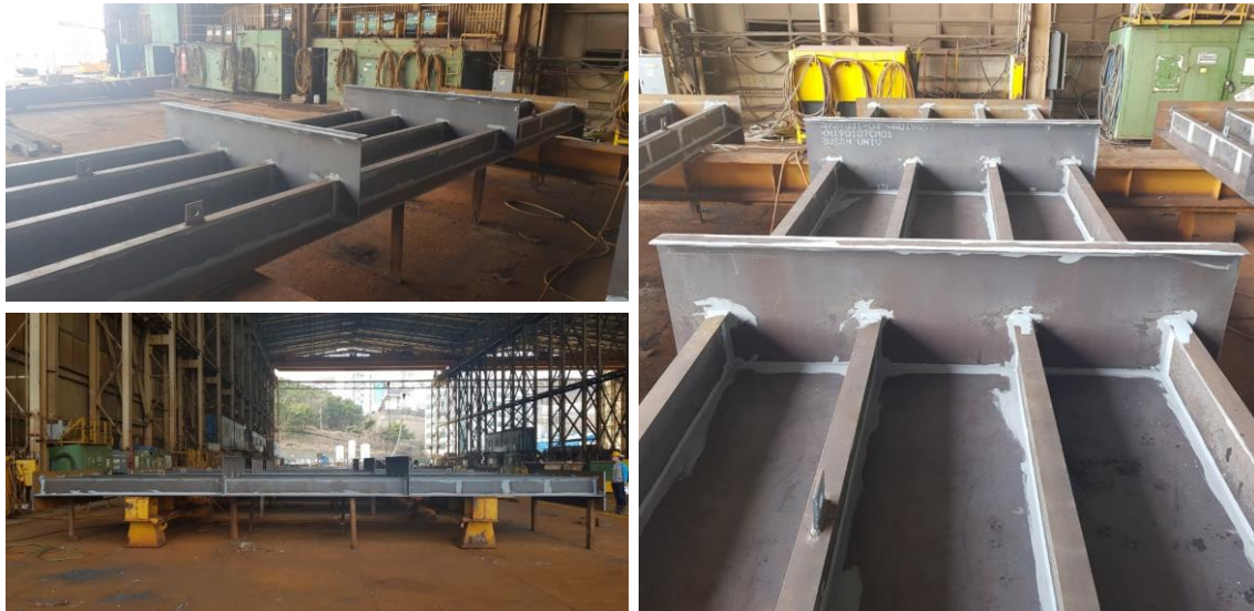
Figure 3. The fabrication of the tested structure at the shipyard.
