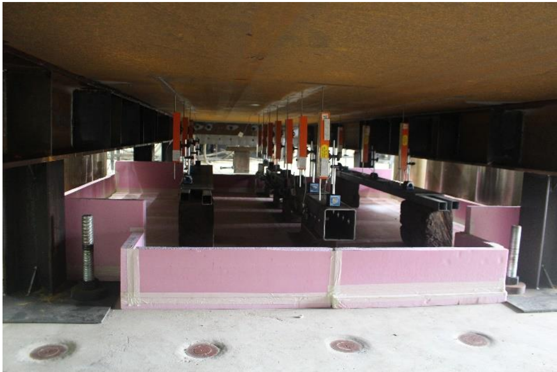
Figure 22. LVDT sensors embodied in the test structure for measuring displacements.
