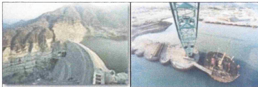
Figure 55. Projects: a. Dam Thysavrou Nestou / Rion – Antirion bridge.
