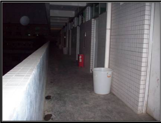
Hallway that leads to workers' dorm rooms
