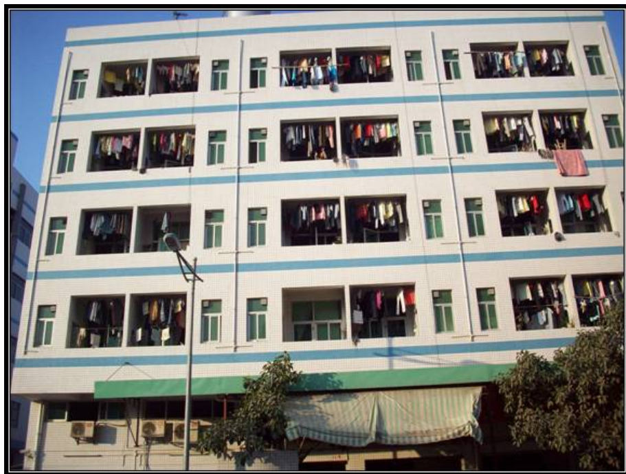
Lever Style Dormitory's exterior
