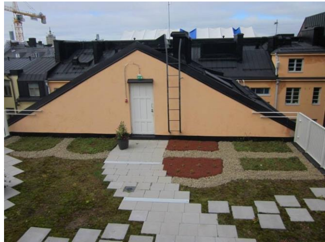
Fig. S2 Vegetated areas and paved paths on the study roof. Moss-sedum vegetation in the front, and newly constructed experimental plots (separated with gravel) in the middle. Photo: Malgorzata Gabrych 2012.
