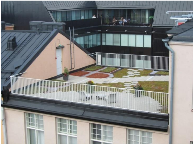
Fig. S1 The study roof. Photo: Ismo Kirves 2012.
