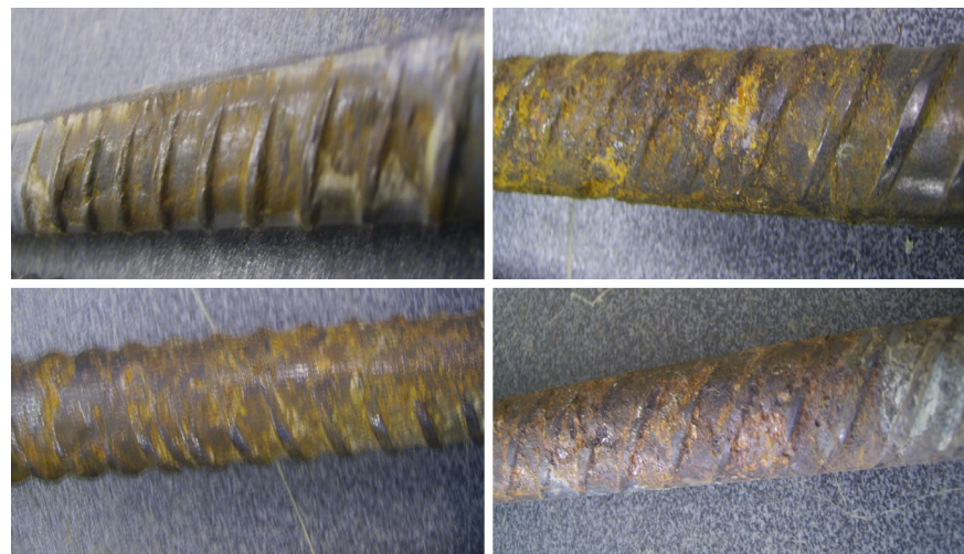
(b) Corrosion of the anodic steel bar (top left is PC concrete and the other ones are AAS concretes)
