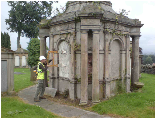
Figure 8. Use of the 400MHz unshielded GPR antennae on a mausoleum, for the detection of internal features.
