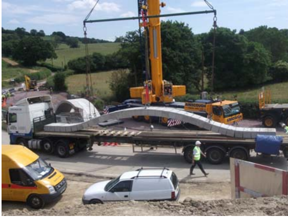
(a) Lifting 13t FlexiArch unit
