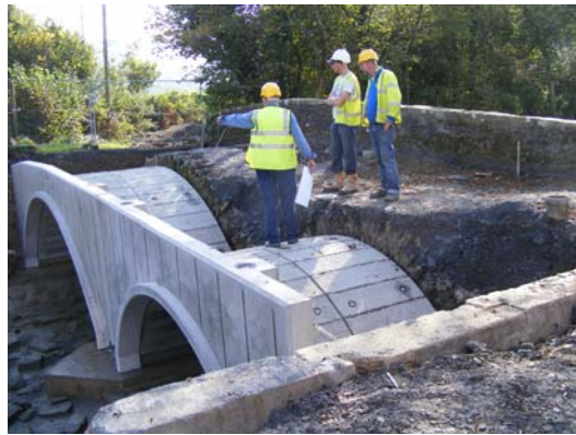
(b) Prior to installation of lean mix concrete backfill
