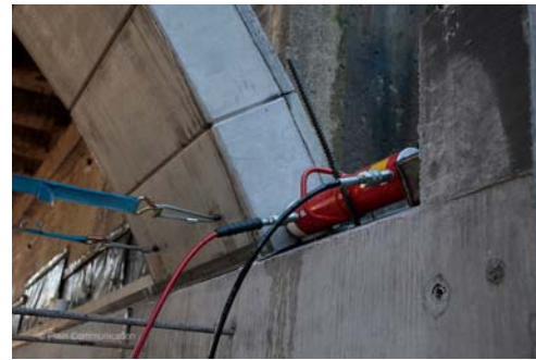
(b) Hydraulic jacking system utilised
