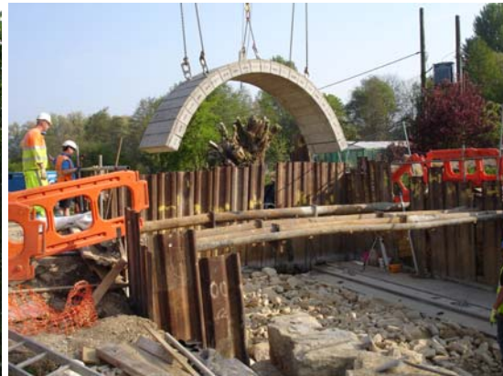
(b) Lowering unit into position
