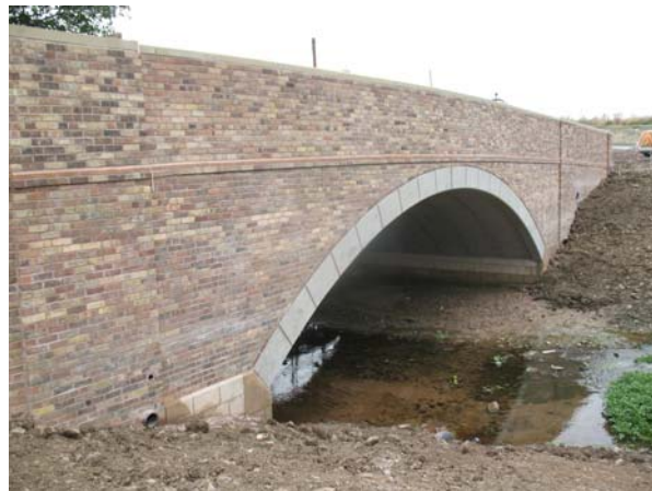
(c) Finished bridge (October 2010)
