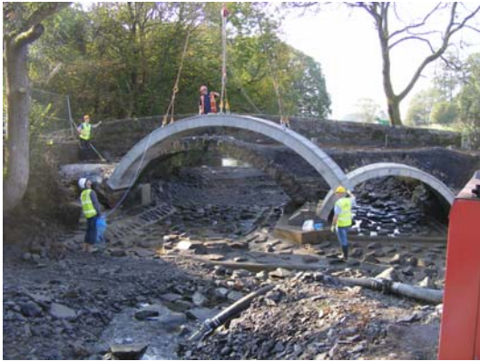
(a) Lowering unit onto sill beams
