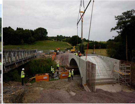
(b) Nearing completion
