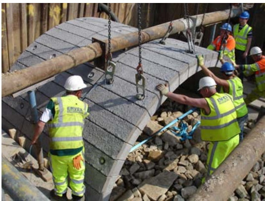
(c) Sliding FlexiArch units under services
