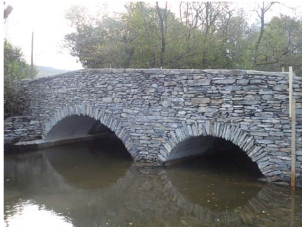
(c) Finished bridge (October 2011)
