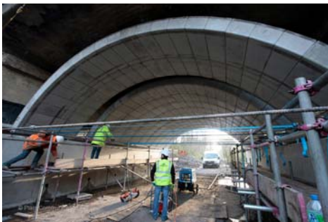
(c) Sliding FlexiArch units along sill beams
