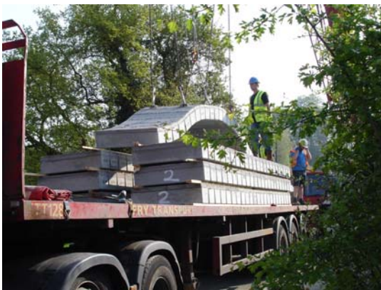
(a) Lifting a FlexiArch unit
