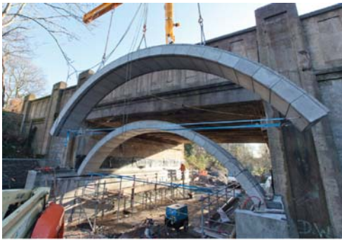
(a) Installing FlexiArch unit on extended sill beams
