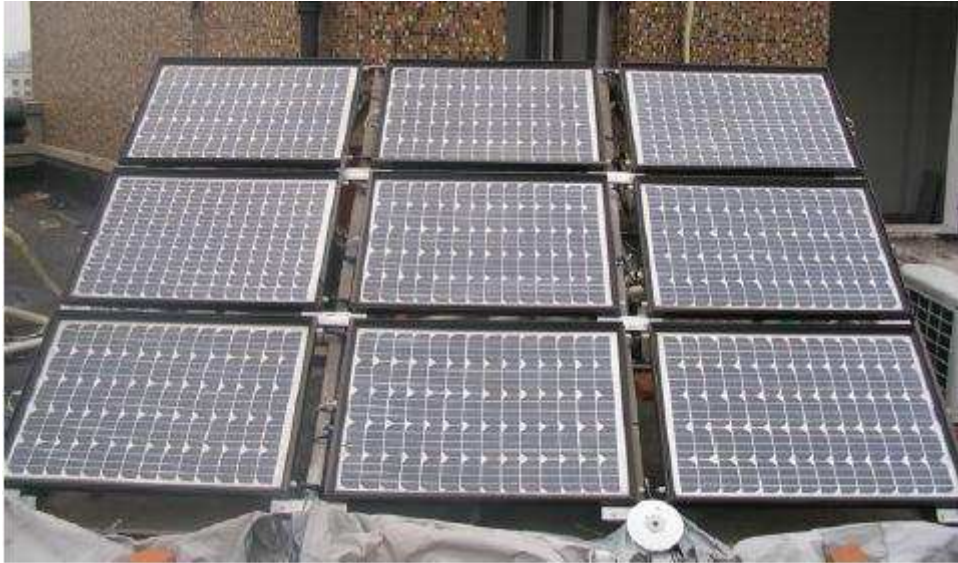
Figure 2.2.10 Refrigerant based PV evaporator modules (Ji et al., 2008)
