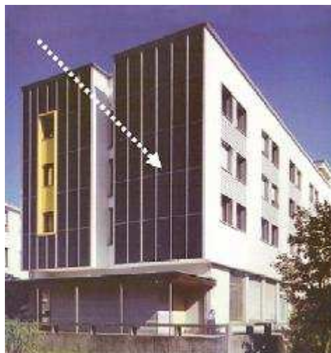
Figure 2.3.3 An illustration of building integrated solar thermal air collector system in a commercial building (Munari et al., 2007)
