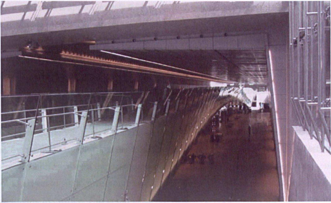
Figure 2.9: Changi Mezzanine Bridge (CMB), Singapore [6].
