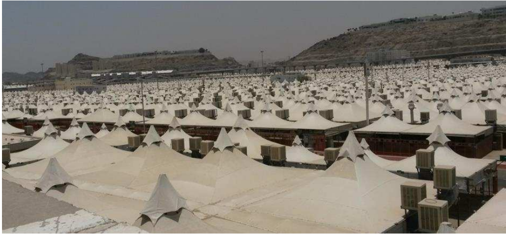
Figure 3.10 Rooftop-mounted evaporative cooler for cooling in pilgrims' accommodations
