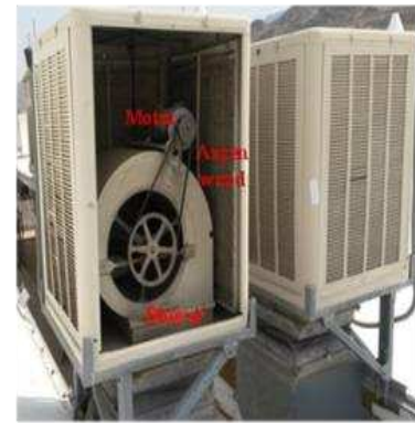
(b) roof-top evaporative cooler unit
