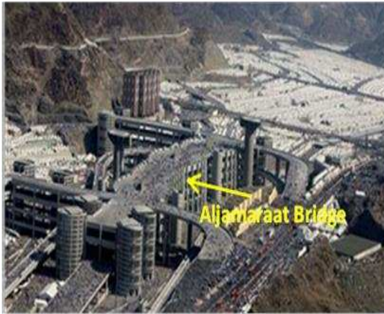
Figure 8.6 (a) Aljamarrat Bridge
