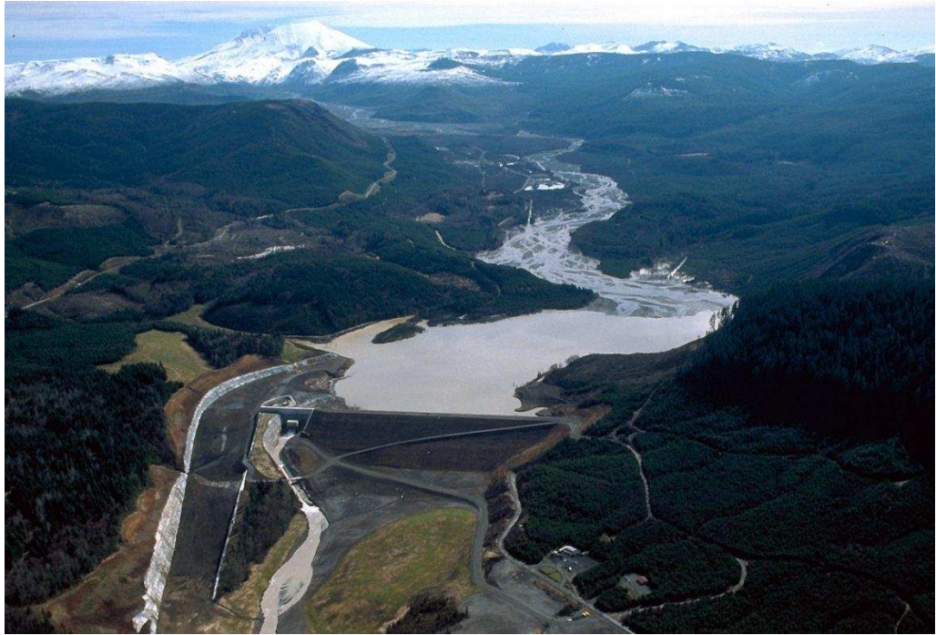
Figure 2.13 North Fork Toutle River Sediment Retention Structure in its initial Phase 1 operation condition, November 1987. Note the pool behind the dam and the flow of water through the structure. Photograph by Bill Johnson (1987).
