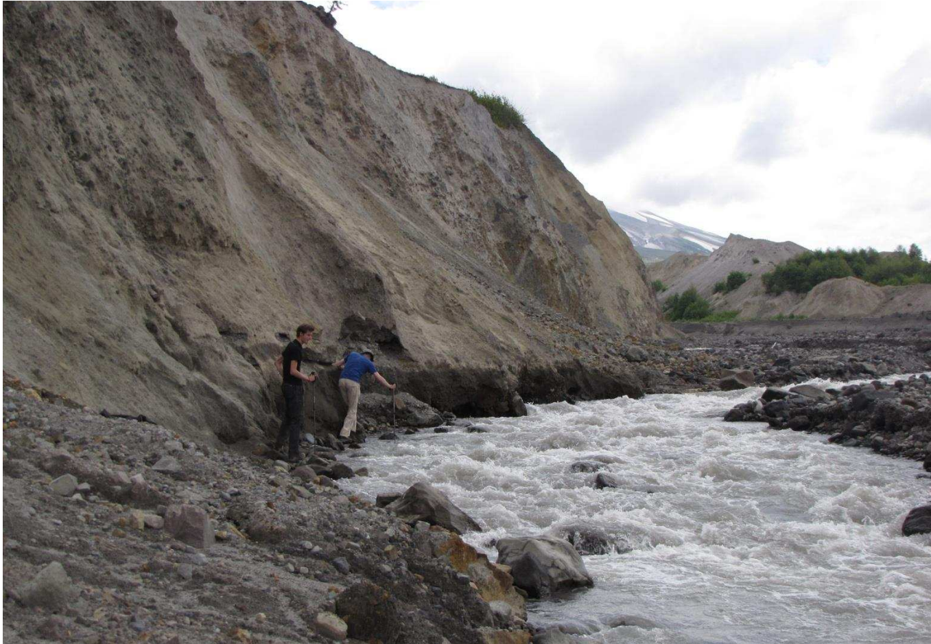
Figure 7.2 Upper North Fork Toutle River near NF120 showing the channel impinging on the toe of its very high and steep bank. Photograph by Colin Thorne (2011). View upstream.
