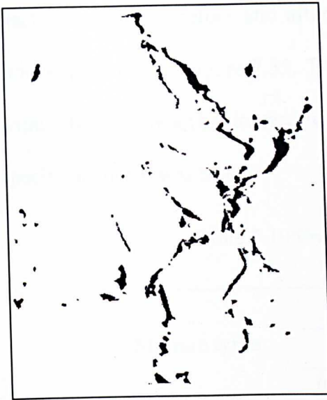
Binary image of cracks
