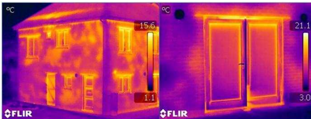
Figure 5-3 - E.On House - Air Leakage Thermal Imaging
