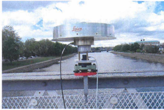
Figure 6-31 The GPS antenna and triaxial accelerometer housed together as one unit, at Bg09.
