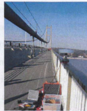
Figure 7-10 Antenna located at Bdg3, secured to the handrails of the bridge.
