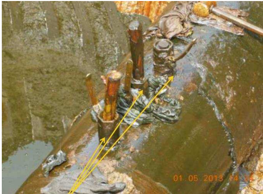
Plate 3-3: Illegal fittings on a 24" Trans Niger pipeline; picture taken on 1 st May 2013 (Shell Nigeria, 2013d).
