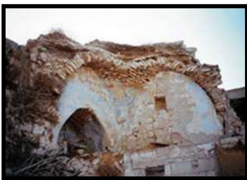
Figure 120: An example shows the materials and contracture of 'Aqid' style in a simple PS traditional house (Type one) in Alkasaba, Nablus.
