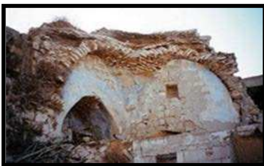
b) Simple house shows the materials and the methods of construction in Alkasaba, Nablus
