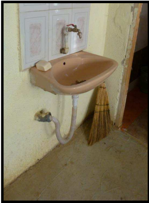
Figure 224: Unsuitable sink for children's scale and use with high point installation
