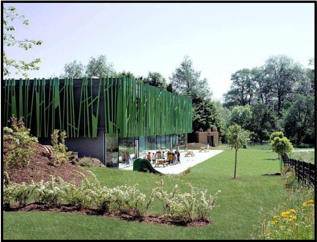
Figure 79: The KG is sheltered from bright sunlight by the external cladding (Photo by Angelo Kaunat, Salzburg).
