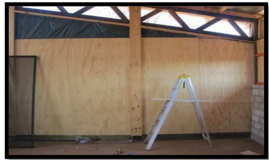
Figure 103: Ply boards to cover the interface walls (UoN, 2011).
