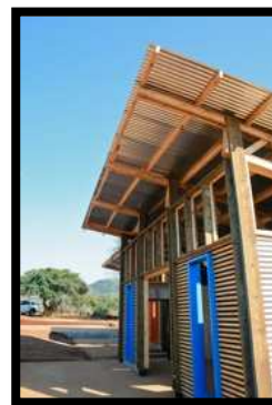
Figure 98: Install the corrugated steel roofing for the classrooms (UoN, 2011).
