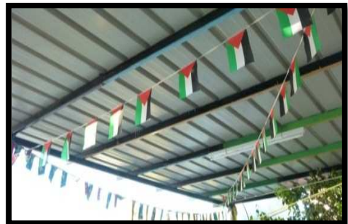
Figure 129: Steel sheets for shading sand area
