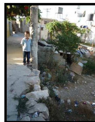
Figure 123: The footpath between the KG entrance and classrooms, A high wall surrounded the (EL) KG, which is a visual barrier (Figure 132)
