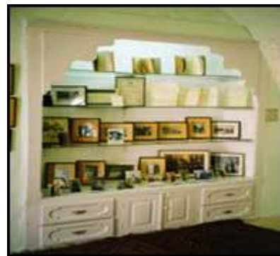
b) The wall thickness has been taken advantage of to install a cupboard. It was originally built as a 'Qaws Elefrash' before converting it later to be used as a cupboard. Located in a bedroom in Bethlehem City.
