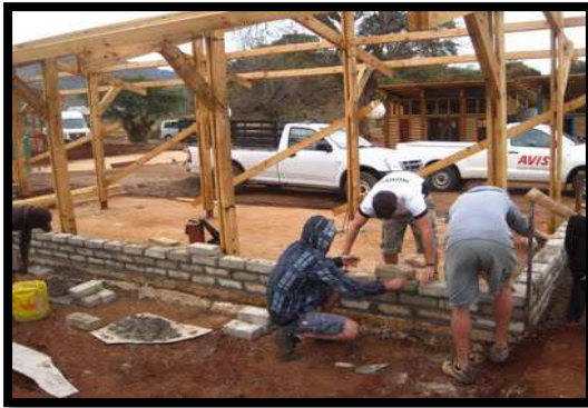
Figure 92: Block walls. Photo by William Holley (Holley, 2011)
