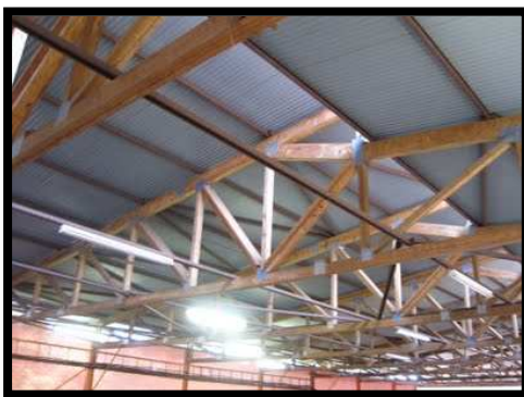
Figure 97: The roof truss. Photo by William Holley (Holley, 2011).
