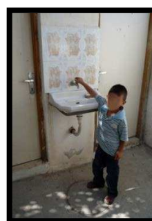
Figure 145: Sinks at inappropriate level for child's use
