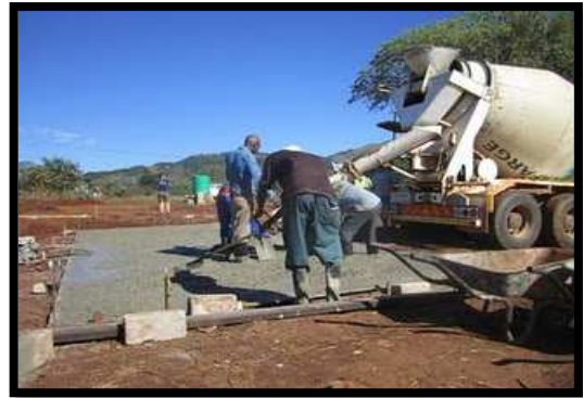
Figure 93: The concrete flat base (Holley, 2011)
