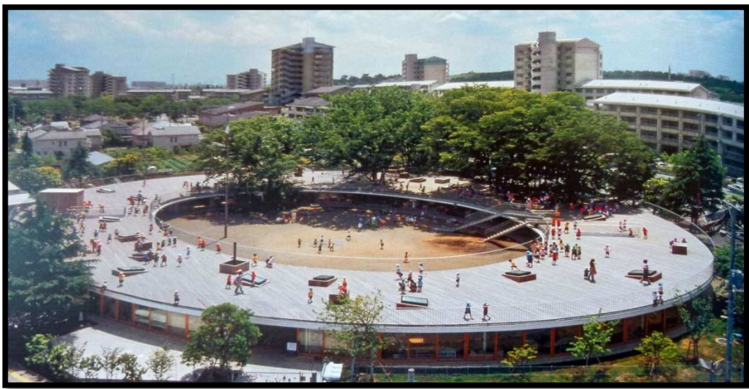
Figure 65 : The roof of Fuji KG in Tachikawa 1,608m 2 , 2007 (DETAIL, 2008)
