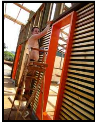
Figure 95: Photo shows painting windows process, and temper cladding for the outer walls (Edmonds, Letter from Limpopo, 2011).
