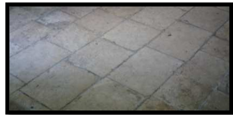
Figure 140: Natural stone floors in classroom No. 3
