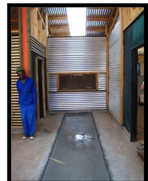
Figure 99: Metal cladding Photo by William Holley (Holley, 2011).
