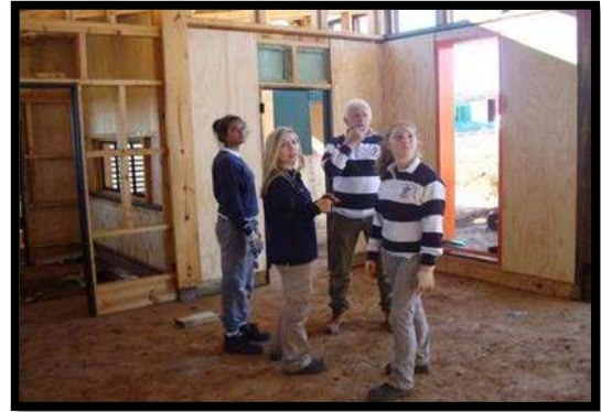
Figure 101: The interior partitions and their wooden structure (UoN, 2011)
