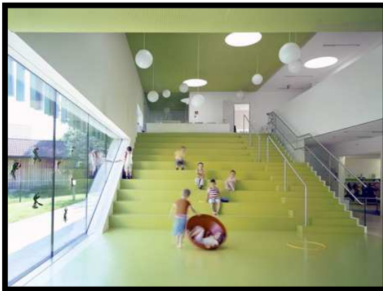
Figure 82: Green lino flooring
