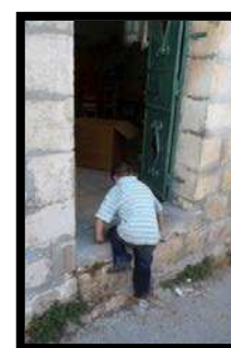
Figure 146: High threshold, class 3
