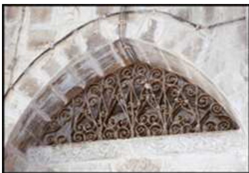
c) An arch vent, which is located above the main door, in Nablus City.
