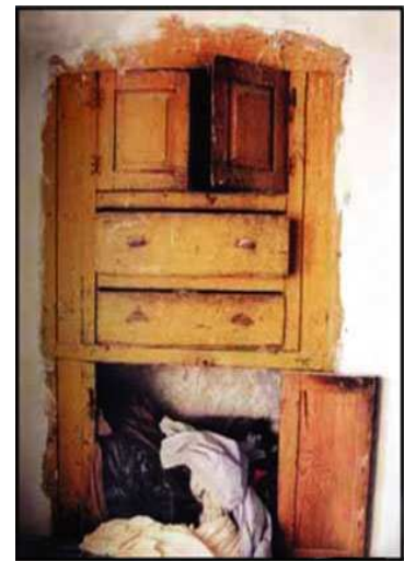
Figure 24: Cabinets in the internal wall
