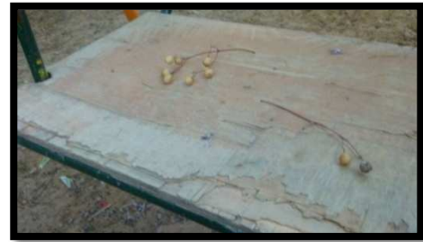
Figure 230: Swing-seat has dangerous sharp edges, and rotten fruits have fallen on seats
