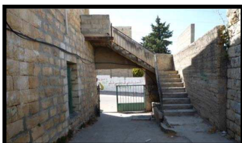
Figure 126: Inside view of the main entrance. The stairs lead to the second floor (a private house)
