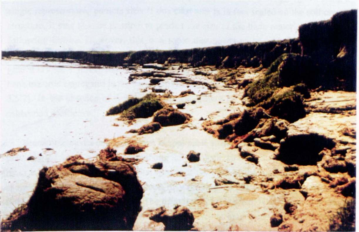
Plate 3.5 Disaggregated Blocks of Cohesive Bank Materials Following Mass Failure of IJssel River Banks, The Netherlands
