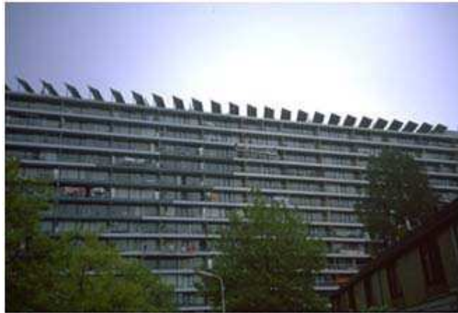
Fig. 2-11. 760 m 2 roof-mounted flat-plate collectors at the Brandaris Building, The Netherlands in 1968 [2.23].
