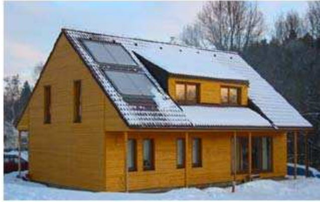
Fig. 2-13. 8.4 m 2 roof-integrated flat-plate collectors at the House W, Czech Republic in 2003 [2.25].
