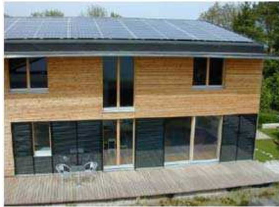
Fig. 2-14. 17 m 2 façade-integrated flat-plate collectors at the Plus Energy House, Austria in 2001 [2.26].
