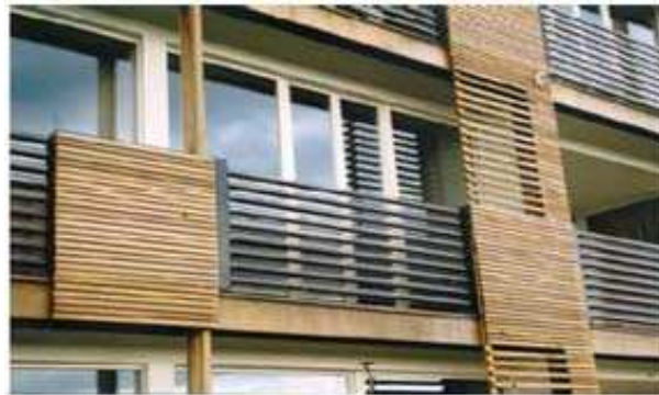
Fig. 2-15. 6 m 2 balcony-integrated evacuated-tube collectors at the Sunny Woods, Switzerland in 2001 [2.27].
