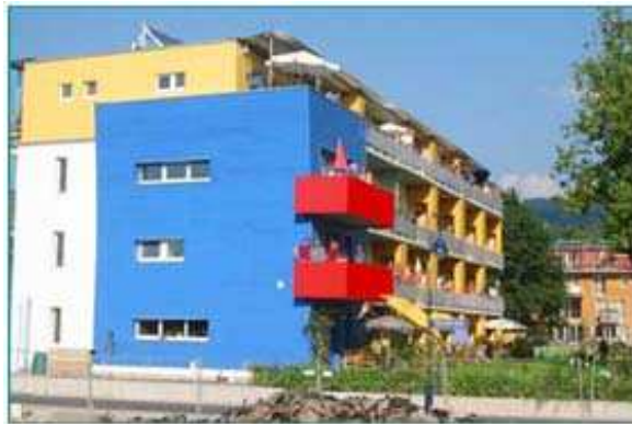
Fig. 2-12. 23 m 2 roof-mounted evacuated tubes at the ISIS Demonstration Building, Germany in 2002 [2.24].
