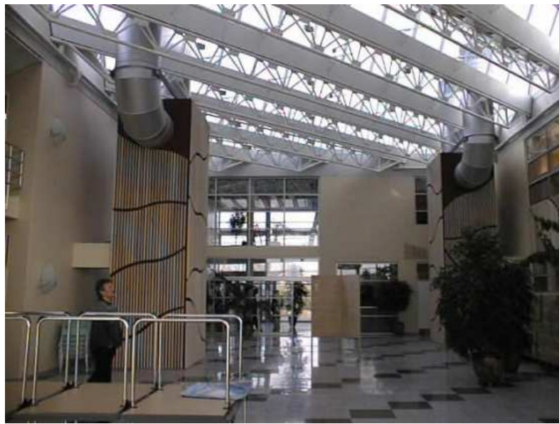
Figure 6:19 The Brundtland Centre in Denmark ( http://www.ecoarchwiki.net/pmwiki.php?n=Projects.TheBrundtlandCentre )
