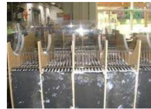
(f) Top water tank
