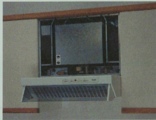
(b) Cooker hood installation
